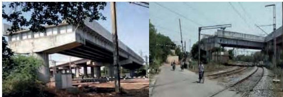
Figure 3.7: East Side (approach was completed but not connected to bridge proper-May 2020)
