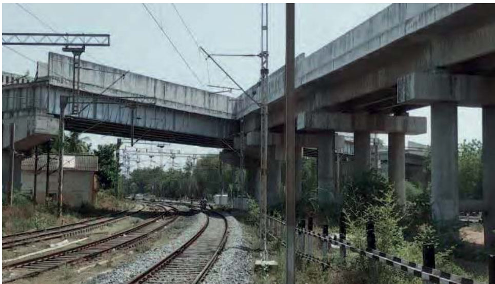
Figure 3.9: West Side (as on May 2020)
