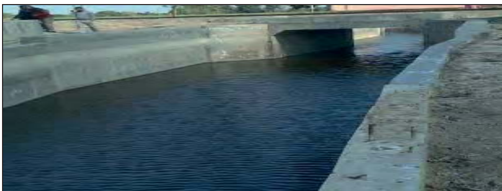
Figure 3.4: LHS at LC No. C-15 (Photograph taken on 6 March 2019)
