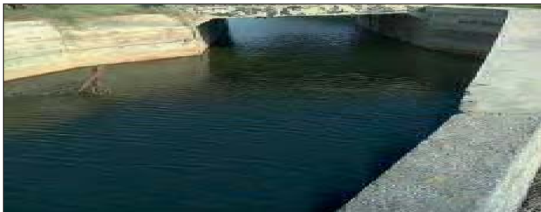
Figure 3.1: LHS at LC No. C-23 (Photograph taken on 6 March 2019)
